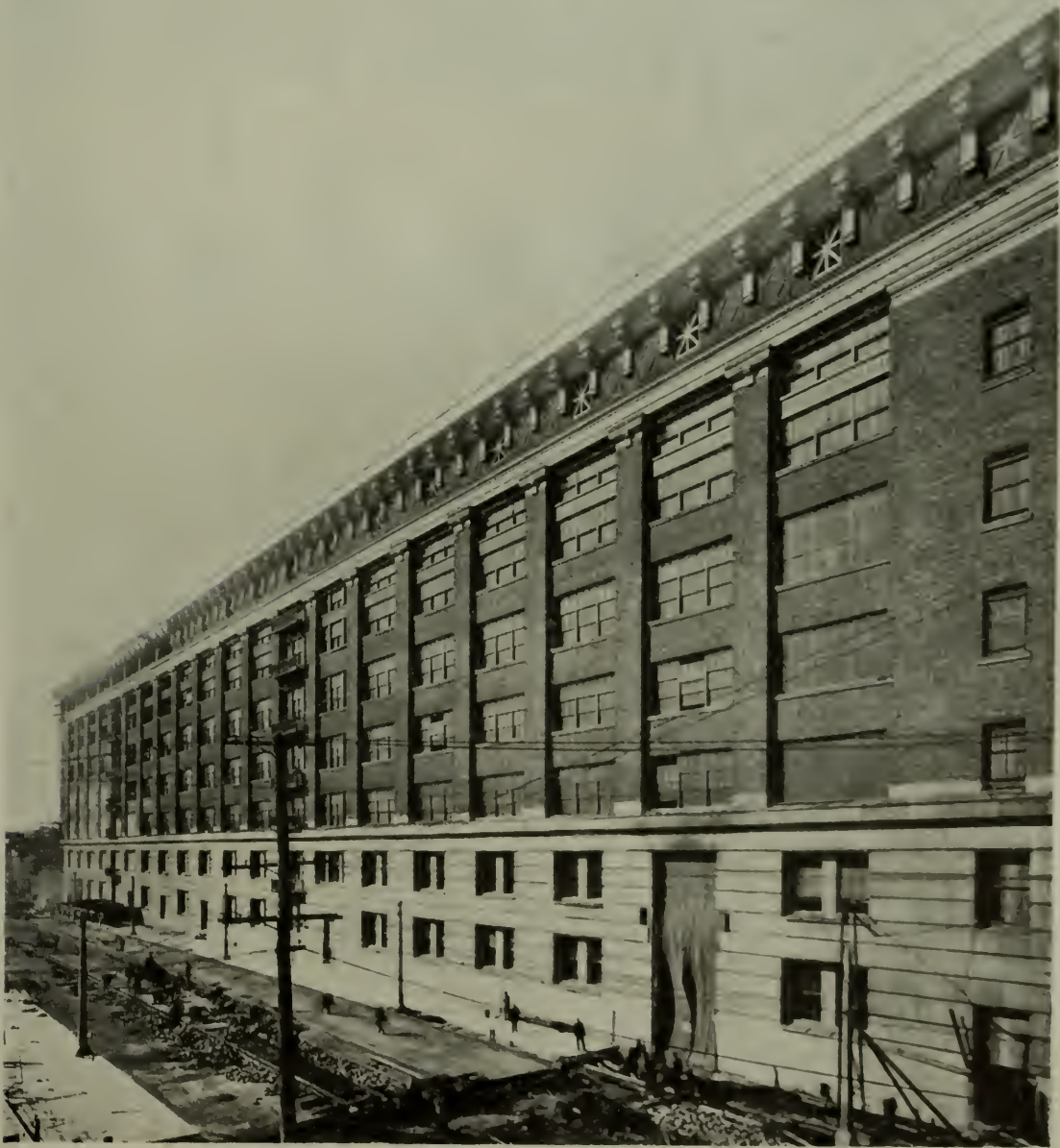
REINFORCED CONCRETE BOTTLING BUILDING, ST. LOUIS: EXTERIOR VIEW ALONG BROADWAY.
